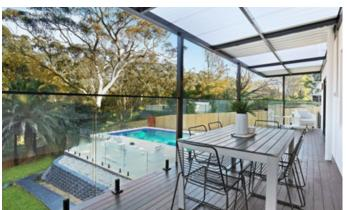
A pool fence's primary purpose is to restrict children's access to the pool area to minimize drowning, but the primary purpose of the barrier is to prevent falls from height or to restrict access for the public. Two different Australian standards cover them. The requirement for a barrier is covered in AS 1288, and the pool fence requirements are covered in AS 1926.
