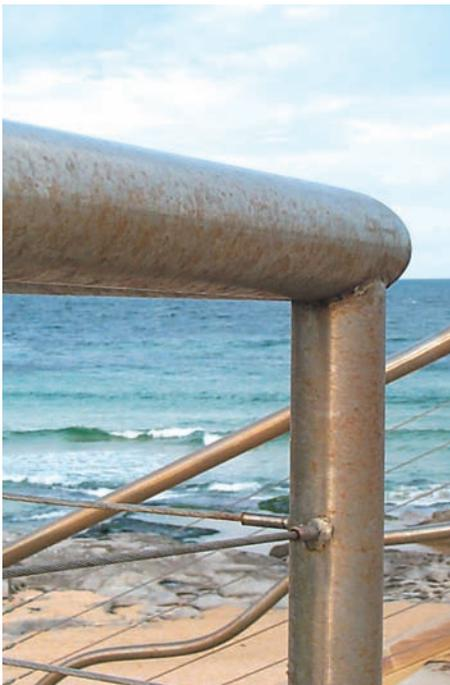
Tea staining of stainless steel in a coastal environment shortly after installation.
